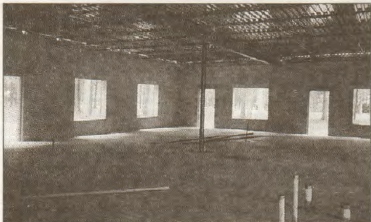
When completed, the simulator complex addition will contain five classrooms. Three of the rooms will be for general purpose use, a fourth for multi-functional applications and the fifth for a crane simulator.
