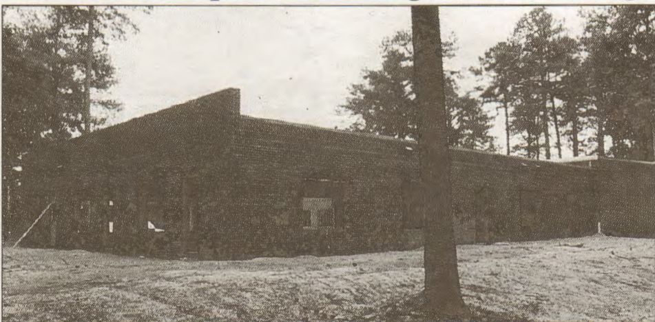
Construction on the simulator complex addition at the Paul Hall Center for Maritime Training and Education in Piney Point, Md., began in mid-April. The facility's exterior has been completed. Construction crews will soon move to the inside to begin finishing the structure's interior.
