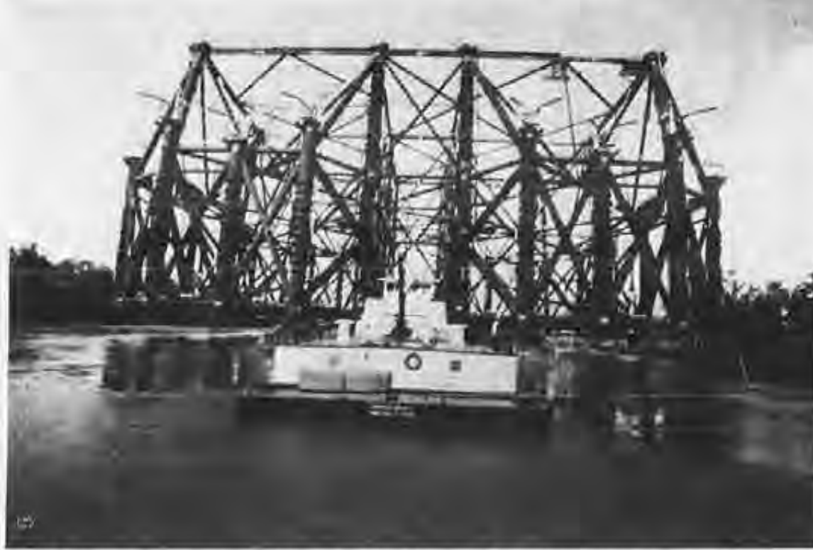
Here's a rear view of the M/V John D. Geary (Orgulf) pushing the first section of the world's biggest offshore oil rig. The rig towers over the trees of Bayou Chene, La. on its way to the Gulf.
