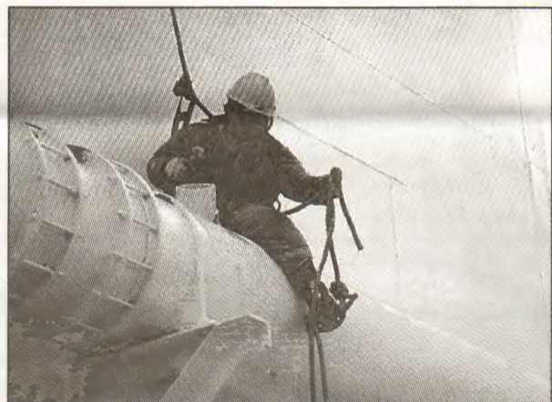
An ATC riding gang member straddles a pipe during maintenance operations aboard the Overseas New York in Cherry Point, Wash.
