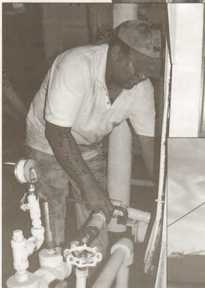
OMU Alfredo Mendoza replaces fittings on hydraulic and cooling systems for the drums.
