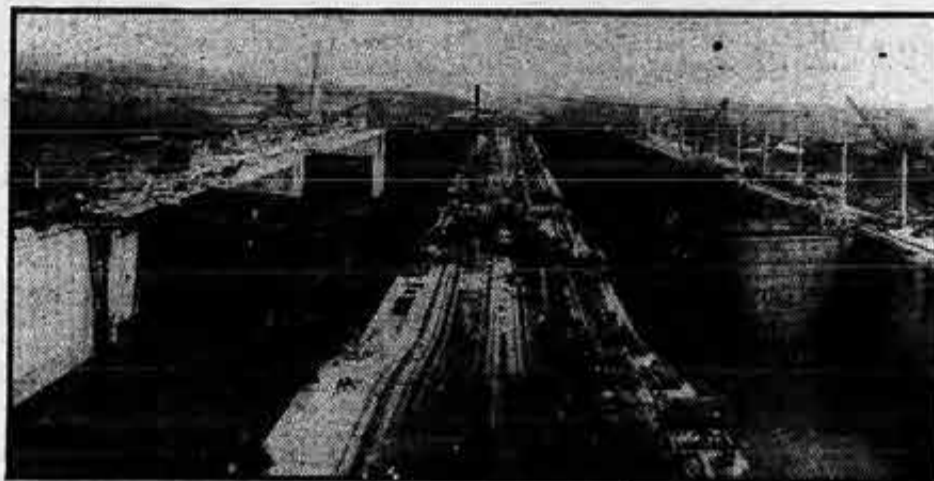
Gatun spillway dam (above) on upstream side, shown under construction, January, 1913. Below are upper Gatun locks clearly showing tracks for the ship-hauling locomotives.
