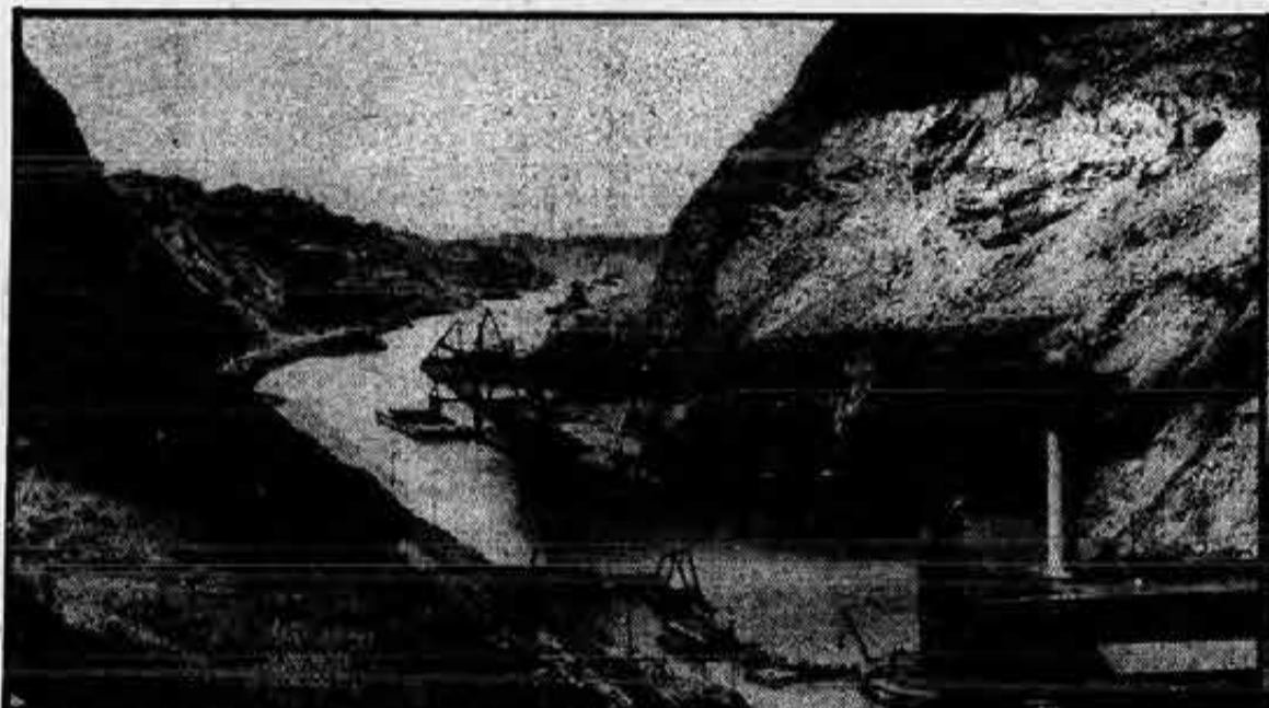
First boat through Gatun locks, a tug, goes under its own steam, September 26, 1913. Vessels are regularly hauled through here by locomotives. Below, dredges clear a slide from the Culebra cut.
