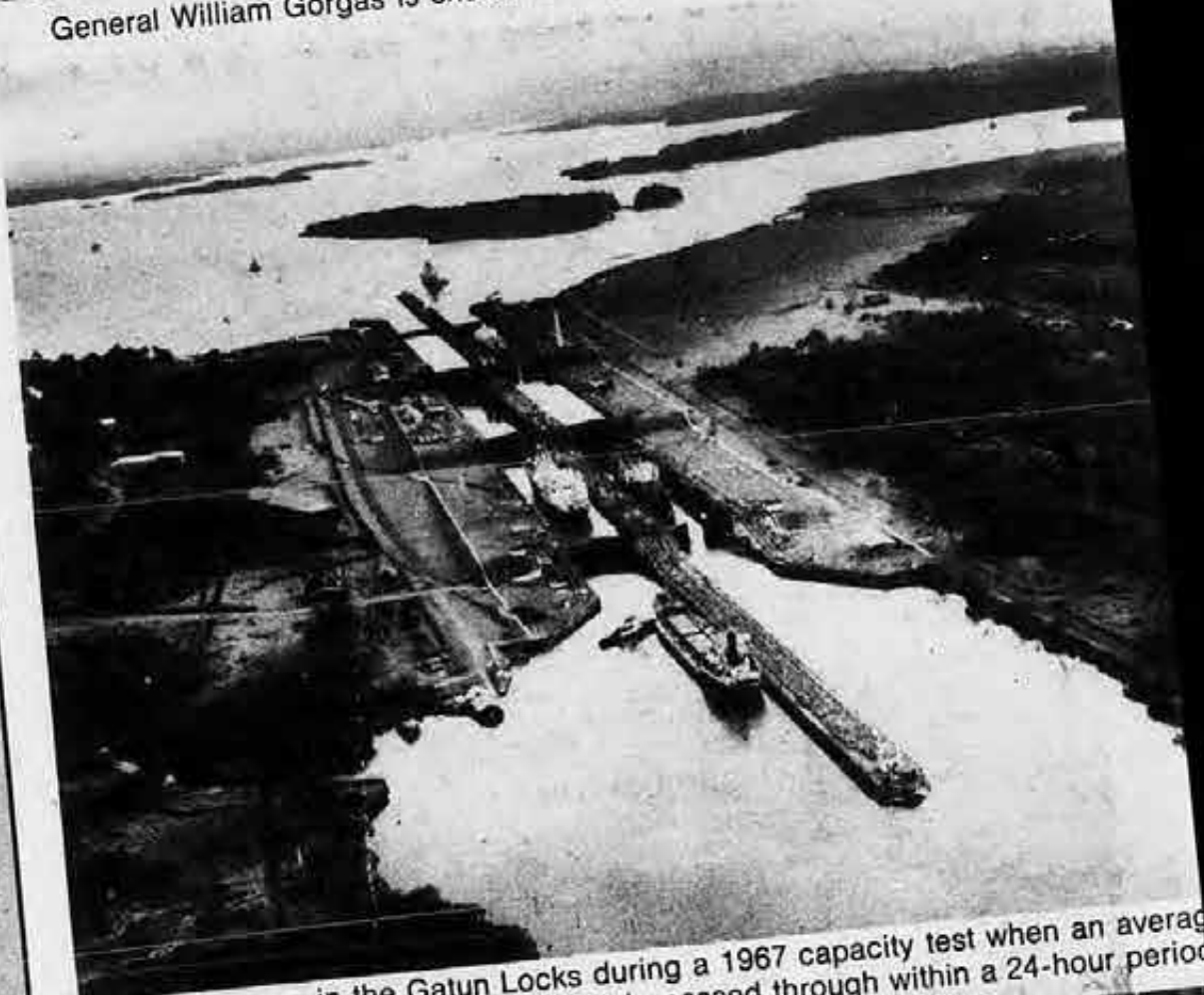
At the Atlantic Ocean side of the Canal are the mile-long Gatun Locks, one of the world's largest poured concrete structures. The two lanes are independent of each other.
