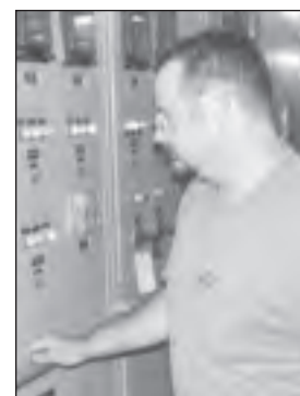
Electrician James Demoui checks gauges aboard the Wright .
