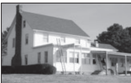
Workers build a back porch on the center.
