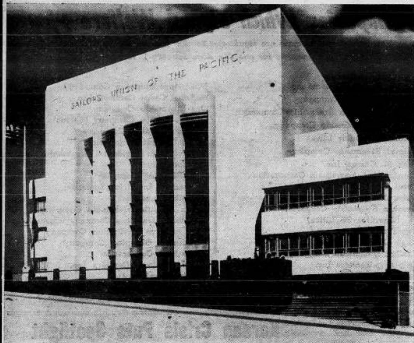
The imposing new SUP Headquarters building fronts on Frisco's Harrison Street. The spacious, well-equipped structure provides practically every type of accommodation sought by its membership ashore. Several SIU affiliates have their West Coast offices in the SUP Headquarters.
