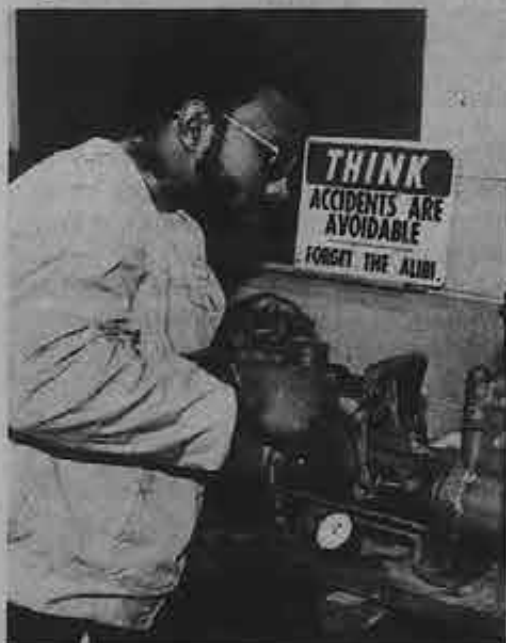
Seafarer Chris Devonish makes a linkage adjustment on a reciprocating pump. Chris ships out of the Port of New York.
