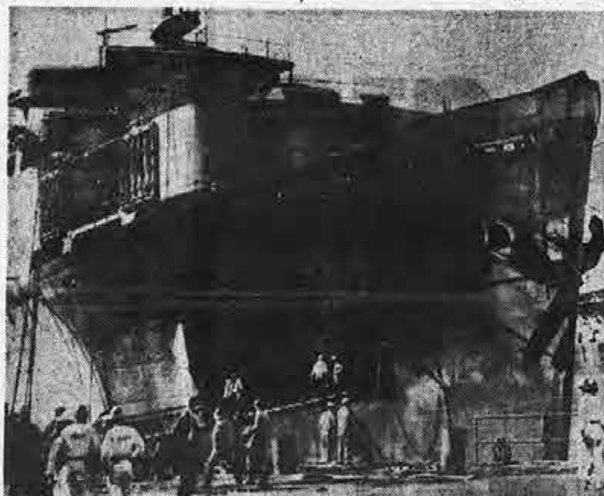
A gaping 15 by 30-foot hole in side of Marine Devil, a C-4 being converted into a trailer ship for SIU Pacific District contracted Matson Navigation, was caused by twin explosions which ripped through vessel at Mobile, Alabama shipyard. No Seafarers were injured but 15 shipyard workers required medical attention. The force of the blast broke windows over a mile away.
