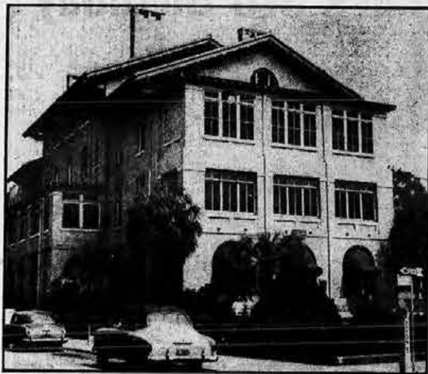
Outside view of Savannah USPHS hospital which will remain open as SIU protests brought change of heart by US Department of Health, Education and Welfare. Hospital will continue to function despite Congress fund cuts in USPHS budget.
