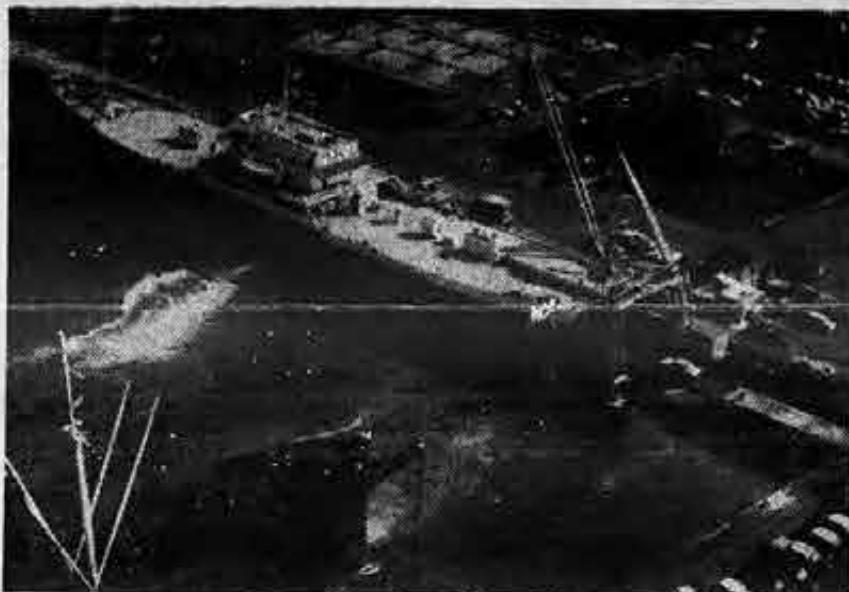
Berthed at Port Newark where this photo was taken, the Floridian has returned to service between Florida and Puerto Rico. Built with an elaborate stern ramp assembly for container use, she will operate as a conventional cargo ship this time out. Palletized freight will account for most cargoes.
