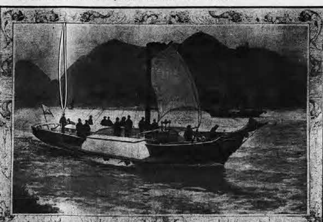
Henry Bell's Comet appeared in 1812 and ran out of Glasgow as a passenger-freight steamer until she was wrecked in 1820. The 30-ton, five-knot vessel had a four hp engine and four paddle-wheels, later reduced to two.
