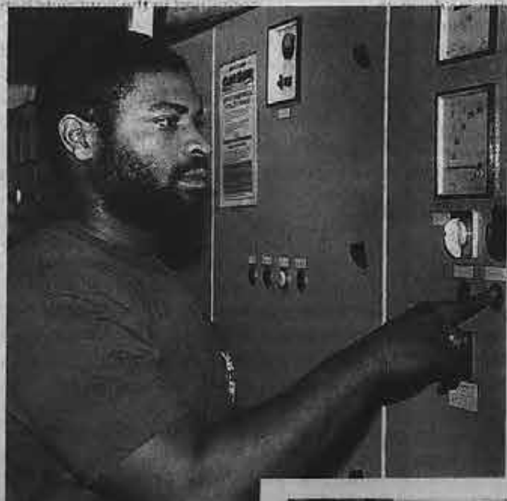
Wiper Roy Jackson turns on the shaft generator on the engine room control board.
