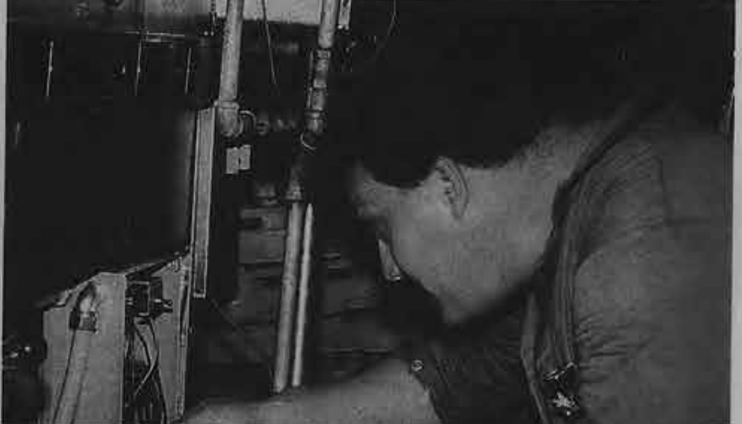
Sometimes the job requires working in cramped spaces as Chief Electrician Edward Mancke discovers while fixing the Independence's dishwasher.
