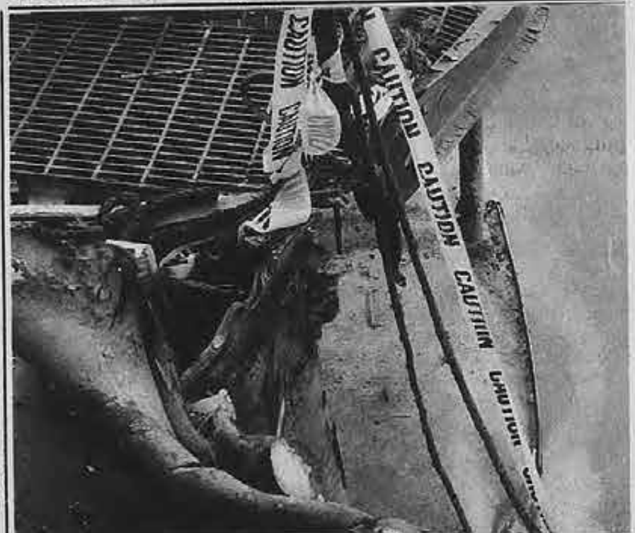
Some of the damage sustained by the Manhattan Island is visible at left.
