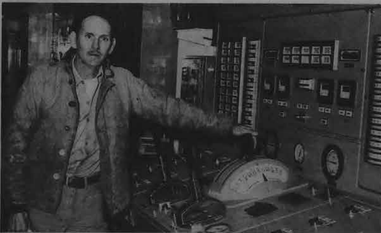
At the controls for the New York's engine room is QMED James Slay.
