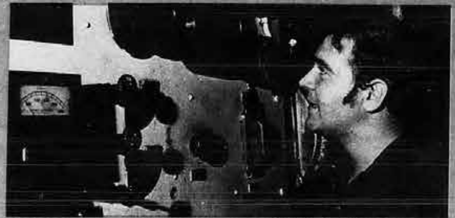
Frank Bakun, who sails as FWT, checks the readings at the boiler combustion control board as the Steel Vendor takes on cargo in Erie Basin. The vessel, a C-4, was preparing for a long voyage to India.
