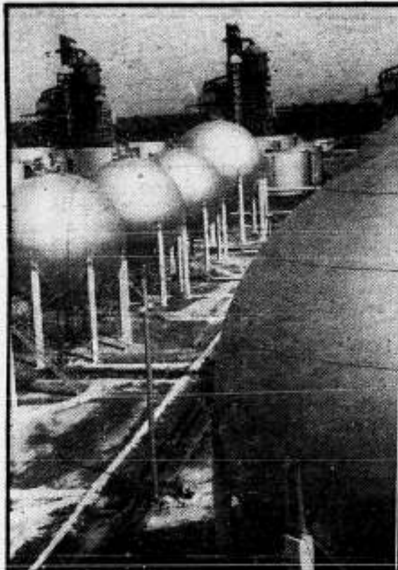
'Crackers' (rear) break up crude oil, pipe it to storage spheres.
