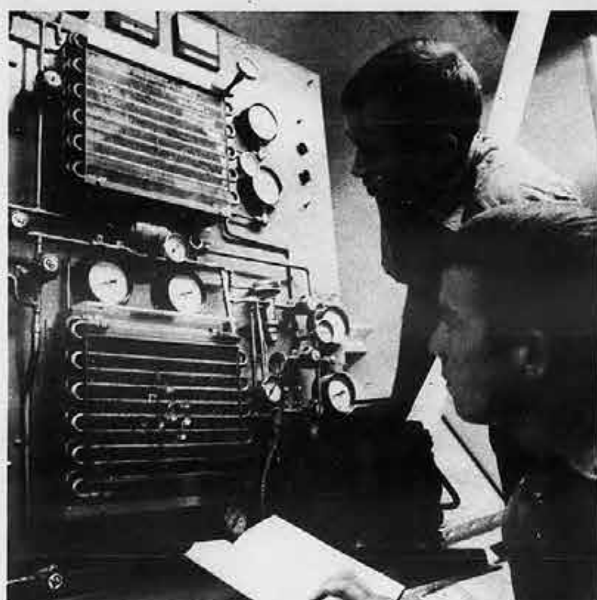
Trainees study a mock-up of a reefer system as part of their two-week course in basic engine department training. Equipment includes all machines and tools that the new seamen will encounter when they board their first ship.
