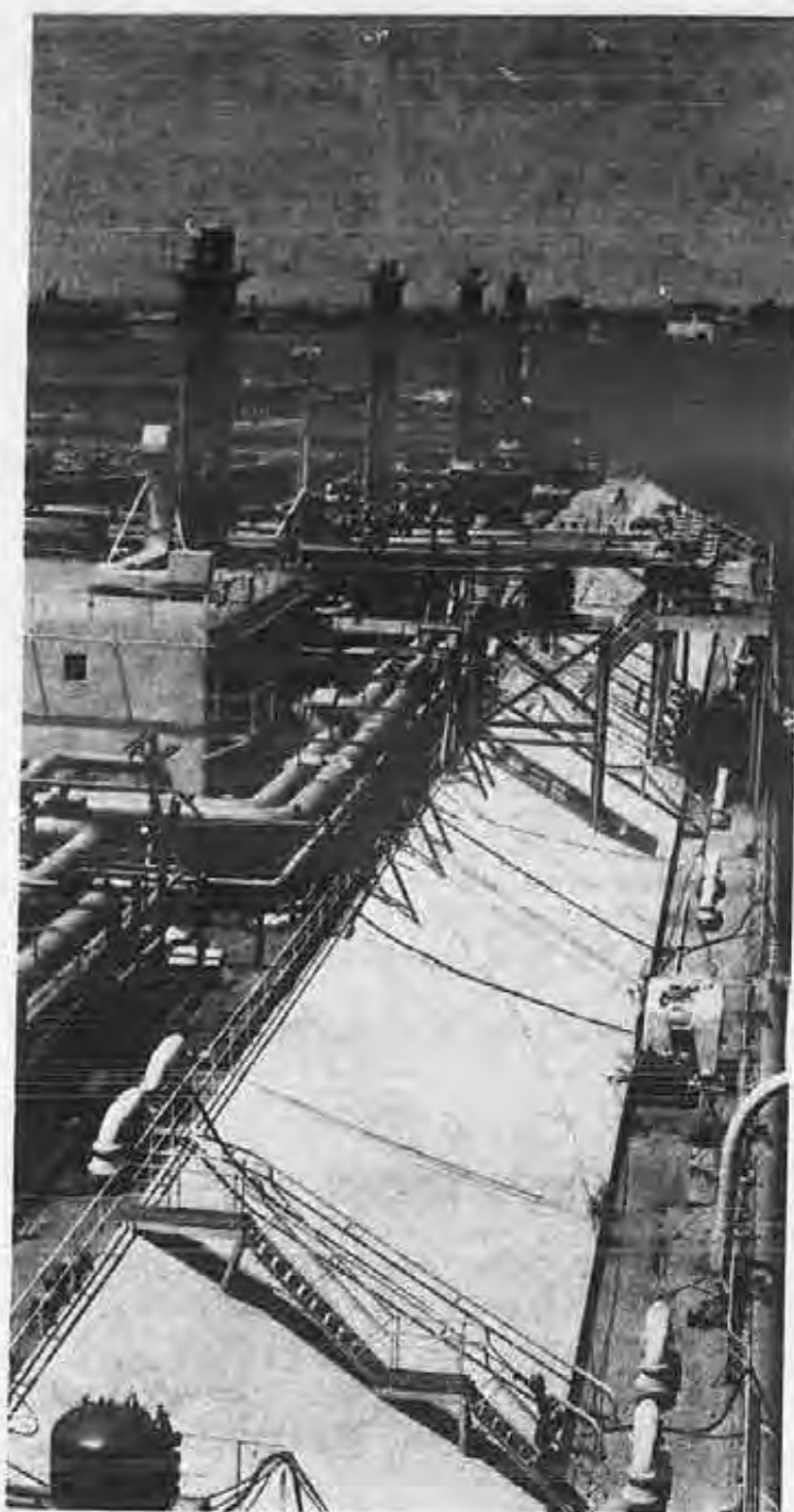
The view from the Southern's bridge shows the top portion of her five cargo tanks. The structure amidships is the Cargo Control Room.
