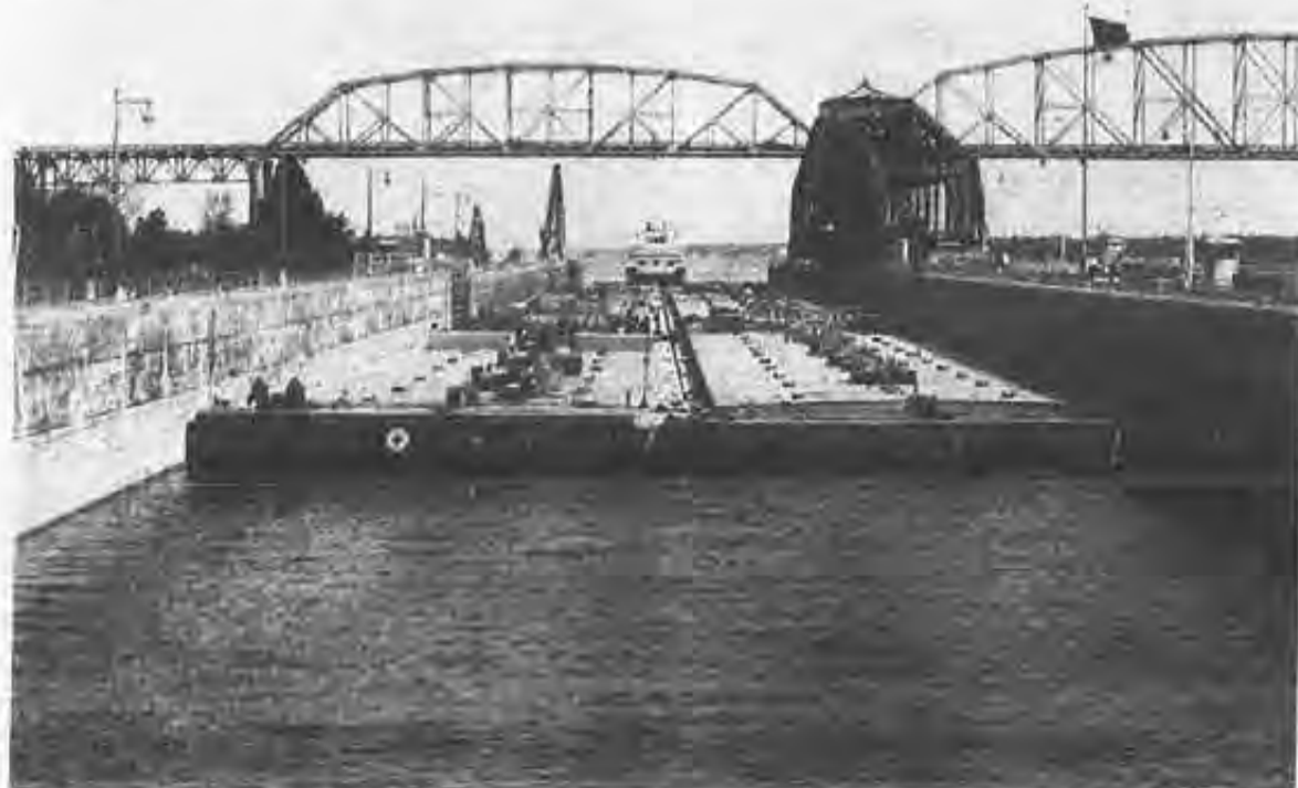
The 600 ft. long Lock 26 at Alton, Ill., shown here, is too old and too small to handle heavy barge traffic at this key point on the Mississippi River. But Congressional delays of legislation which would allow a new, larger lock—along with inland user charges—have been almost as long as the back-ups caused by the old lock.
