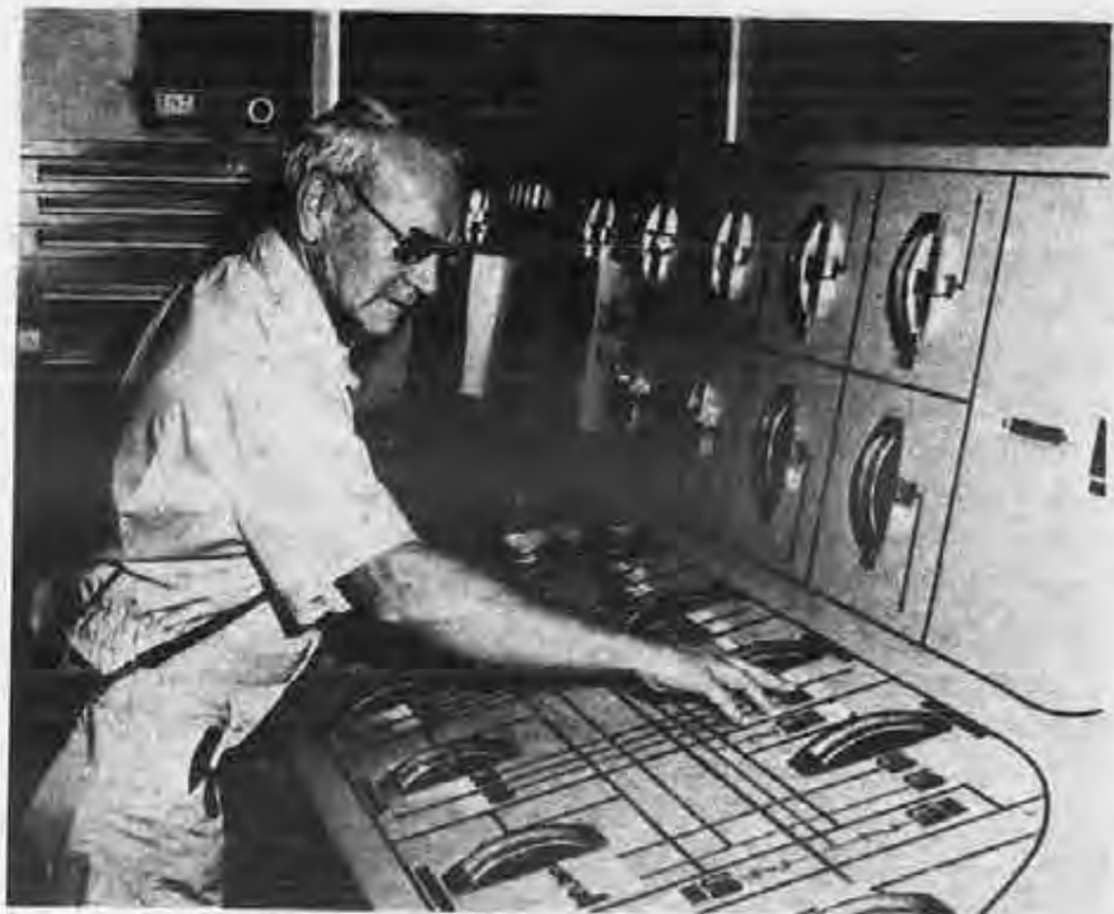
Quartermaster R. E. Ramage opens one of the forward ballast tanks with the pressing of a button on the Ballast Control System Console which is located inside the Cargo Control Room.
