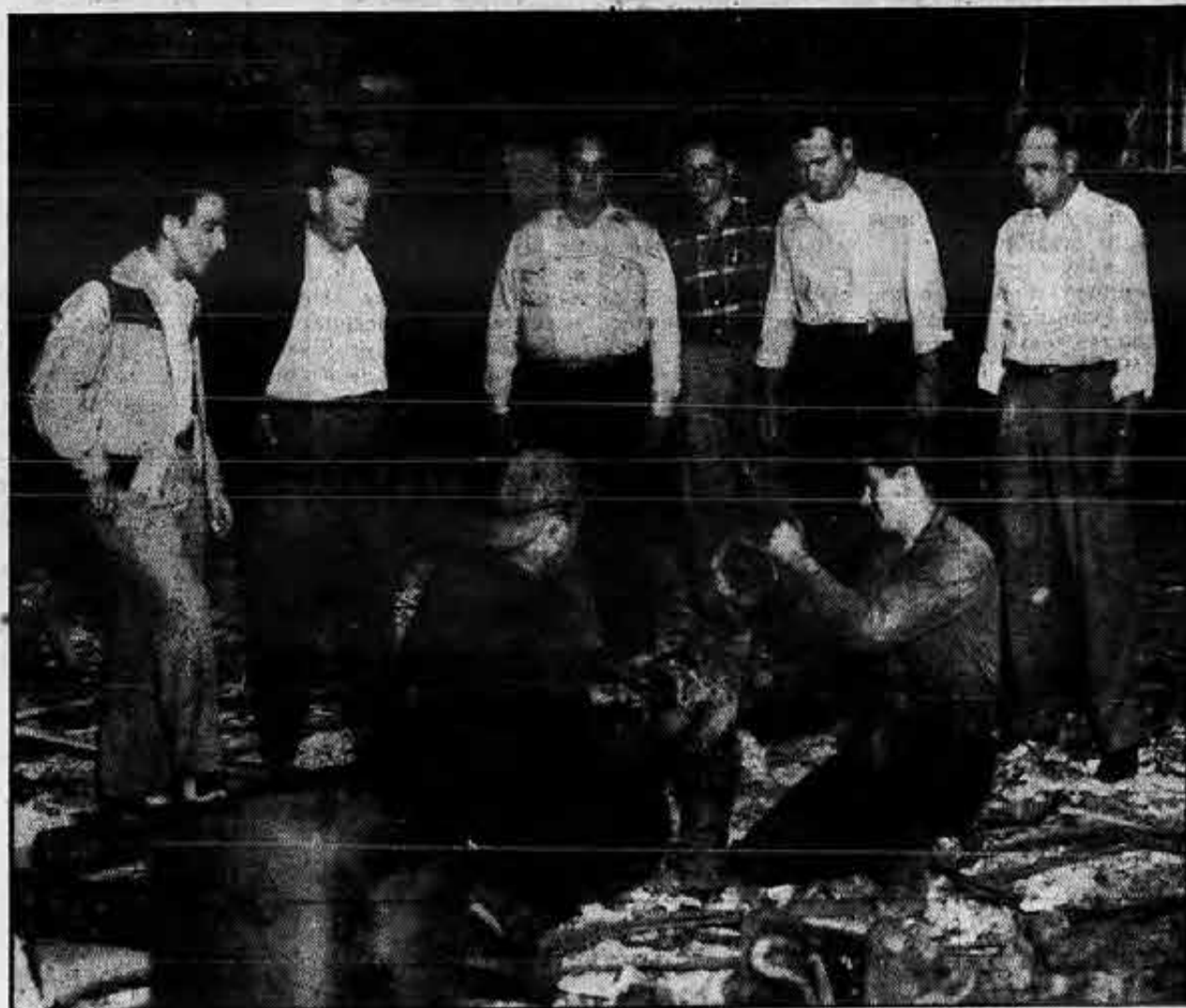
Seafarers are interested spectators as work gets under way on new Baltimore hall. Left to right are: Smoky Messinger, electrician; Al Stansbury, patrolman; Gil Semeff, bosun; Jim Morgan, OS; Pat Robertson, OS, and Bill Addison, oiler. Barring delays, work is slated for completion by Christmas.
