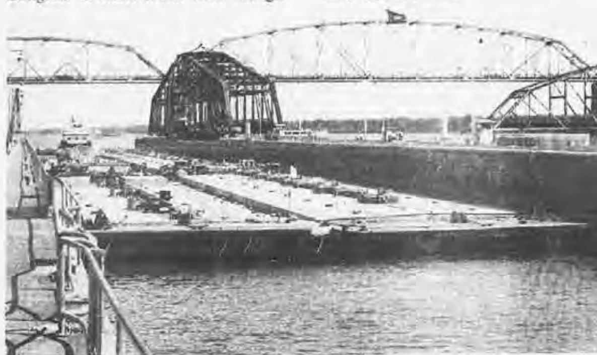
The long-fought battle to get Locks & Dam 26 restored finally ended with some good news and some bad news. Though the facility will be replaced, Congress tacked on an amendment to the bill authorizing funds for the renovation which imposes a fuel tax on inland waterway users.
