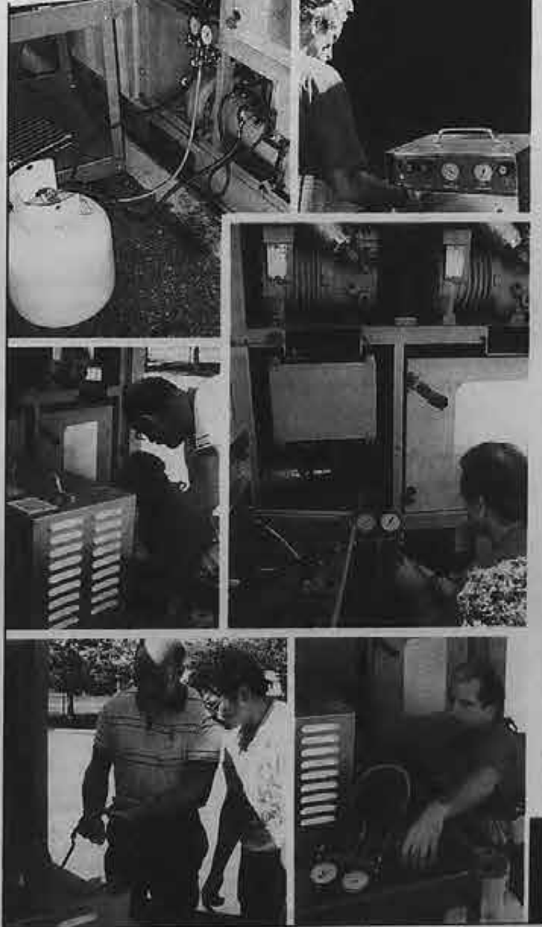
Seafarers at the Lundeberg School conduct an exercise removing refrigerants from a large refrigeration unit. Above is a sample of the card a Seafarer will receive upon successfully passing various or all sections of the exam.
