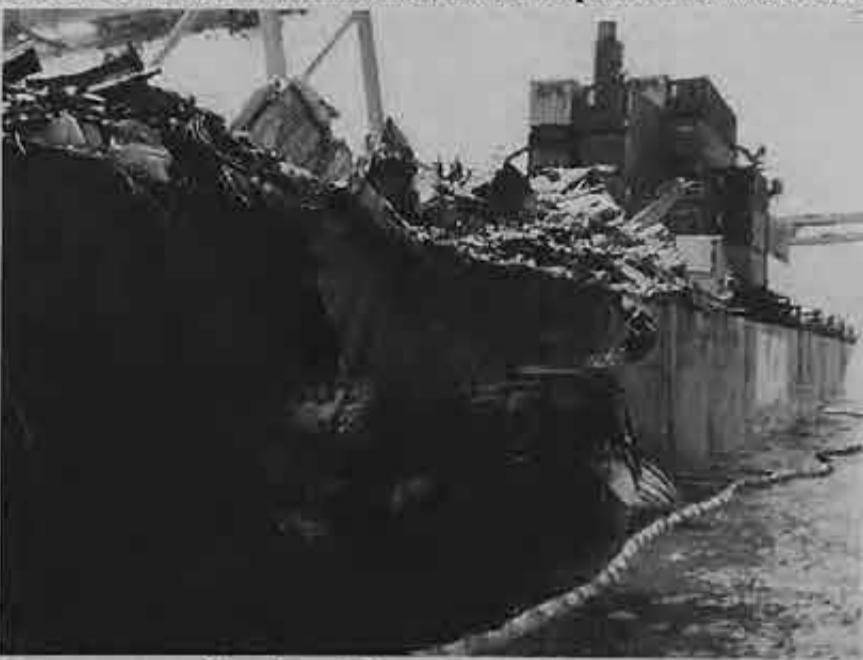
Damage caused by the collision with the Hanjin Hongkong can be seen in this photo of the President Washington , photographed by Asst. Cook Ernesto Billanuba.
