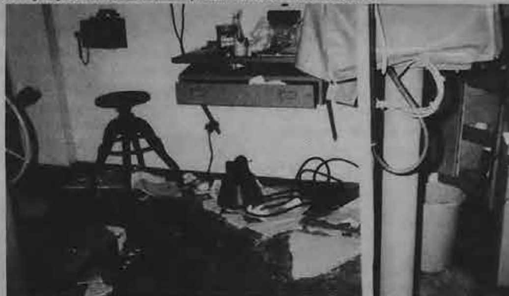
This photo of the Cove Ranger's wheelhouse shows some of the force of the explosion which shattered parts of the ceiling and walls. Fire damage was severe in other parts of ship.
