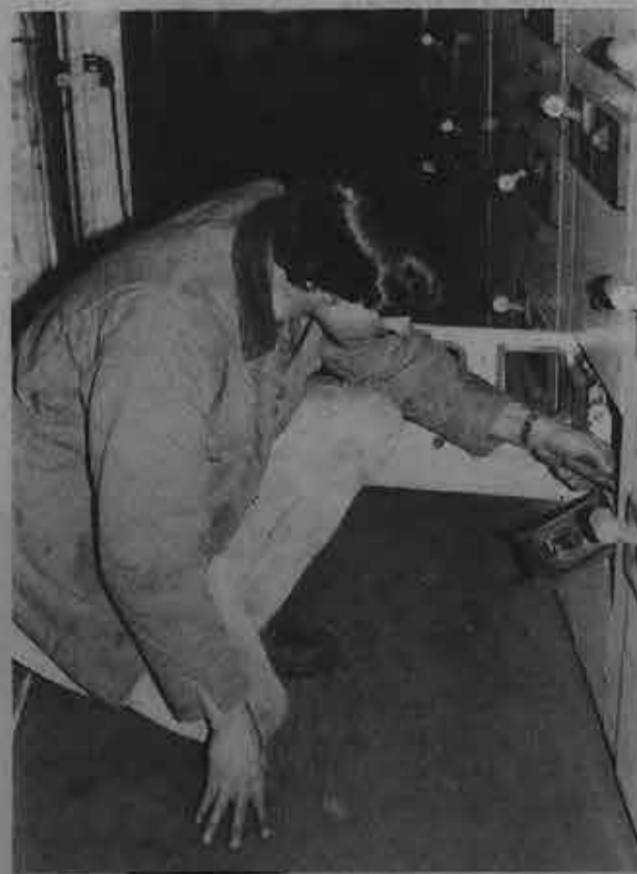
Dan Oberle, electrician, gives a few final turns of the screwdriver aboard the Indiana Harbor .
