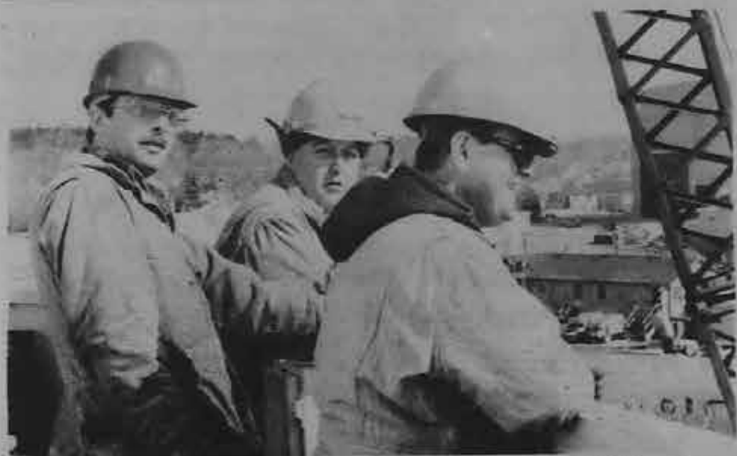
From aboard the H. Lee White , Wheelsman Louis Diehl (l.), shipyard worker Joe Feld (center) and Watchman Dwayne Witt watch the activities on shore.
