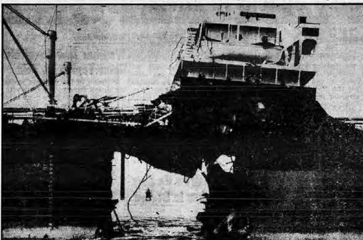
The Tanker Ticonderoga limps into Los Angeles Harbor with gaping hole blown in her middle by mysterious explosion at sea. Inbound from Honolulu, the tanker came in under her own power, with no injuries reported in the mishap.
