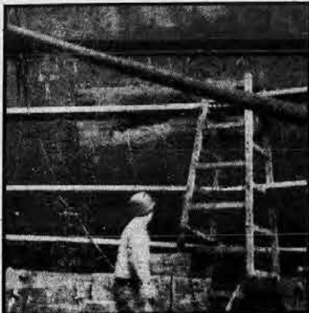
Local shipyard worker in Kobe, Japan, notes the deep gash in the side of the Greece Victory, (left), before complete repairs were made in the Japanese port. Scotty Chisolm, (right), goes over the side in his diving gear to inspect the hull of the ship in its Port Chicago, San Francisco, berth, before the vessel continued on its run with a 10-foot steel patch on its side.
