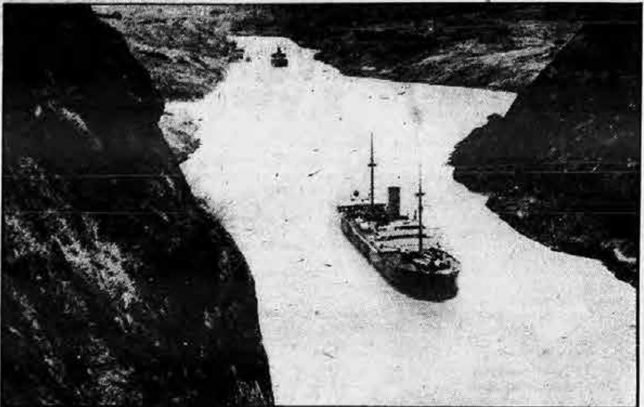
View looking north (toward the Atlantic) at the Gaillard Cut, where the Panama Canal cuts through the hills of the Continental Divide. Contractor's Hill, at left, is where a huge crack threatens a landslide which could close the vital waterway. Some 2-3 million tons of dirt and rock will be removed from the top of the hill, which is 325 feet above the canal level.
