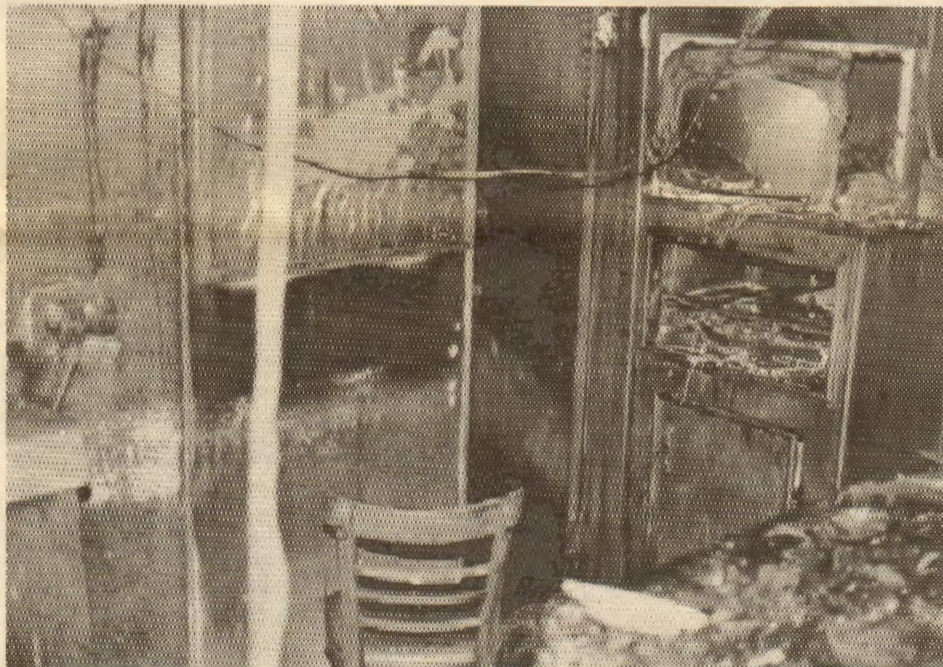
The fire spread from the engine room, and the flames and the heat caused considerable damage throughout the tug.
