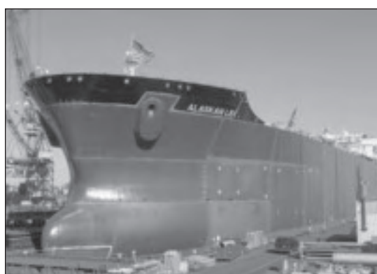
The Alaskan Legend (pictured during construction early last year) is the newest double-hulled tanker in ATC's fleet.
