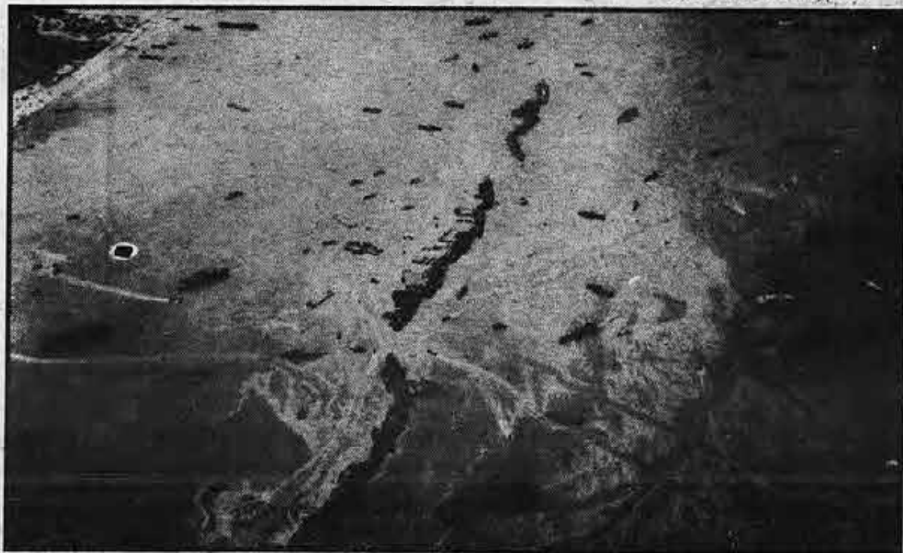
A line of Liberty ships (dark chain running through center of photo) form a man-made breakwater off the Normandy Coast shortly after D-Day, 10 years ago. Ships were scuttled to afford calm surf
