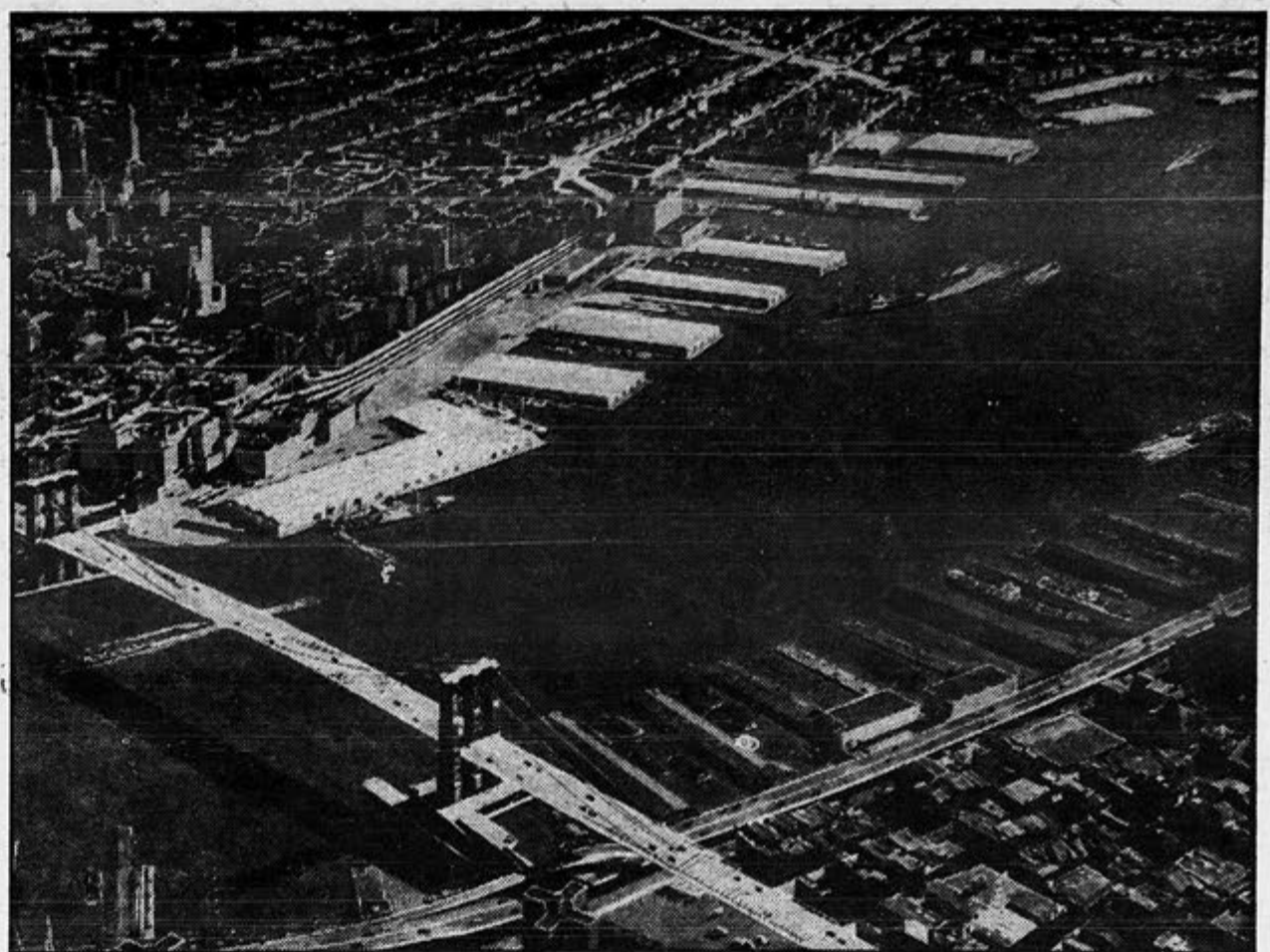
View looking south from Manhattan side of Brooklyn Bridge shows two miles of Brooklyn waterfront as it will appear upon completion of seven-year, $85 million Brooklyn-Port Authority pier development program. Twenty-six existing narrow, obsolete piers will be replaced with ten modern structures and another will be completely rehabilitated. The development will provide a total of 25 modern ship berths.
