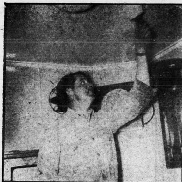
Overheads on the DeSoto get the onceover with a new coat of paint supplied by member of the Waterman shoregang in New York. Seafarer A. Danne took the photo.
