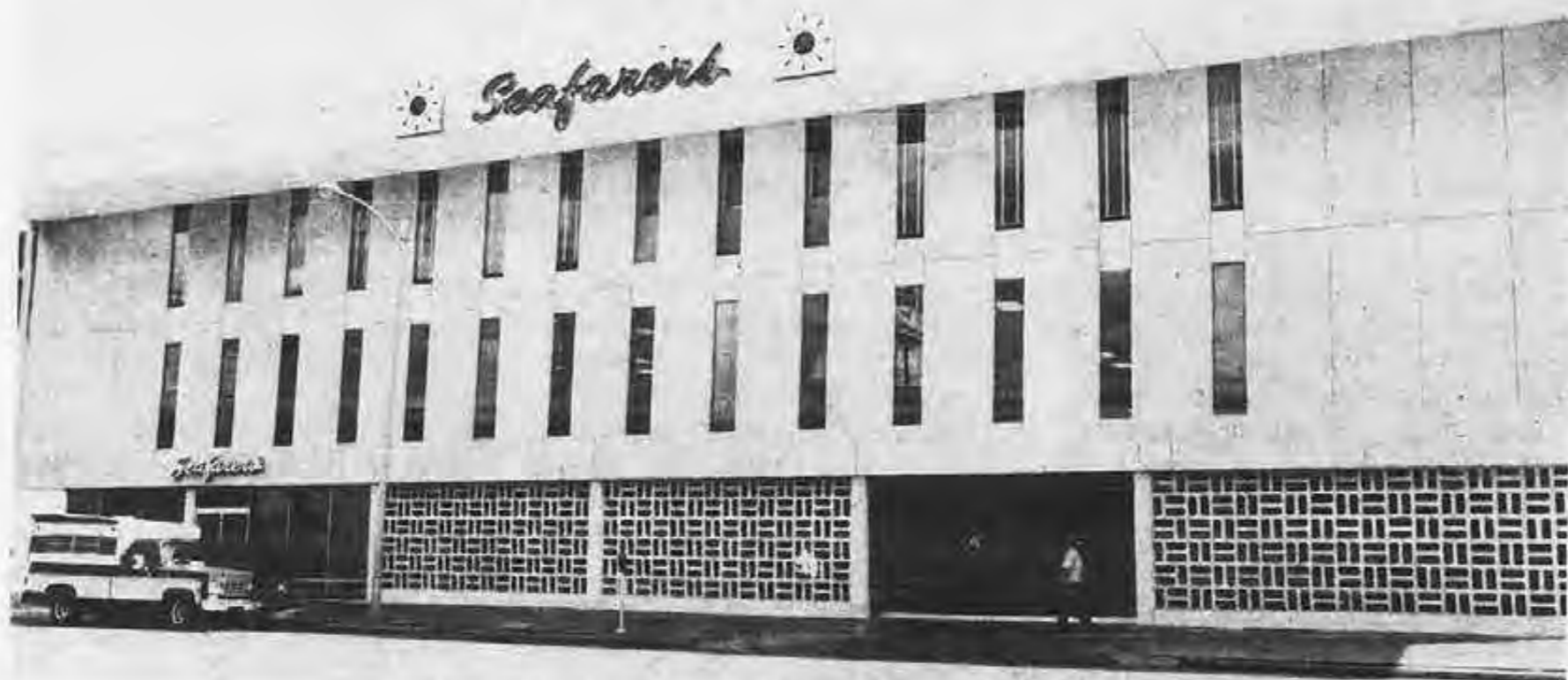
An outside view of the new Houston Hall at 1221 Pierce St.
