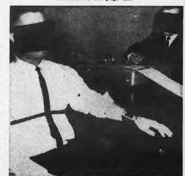
"Lie detector" measures pulse and breath rates. Experts have found the devices highly inaccurate and unreliable.
