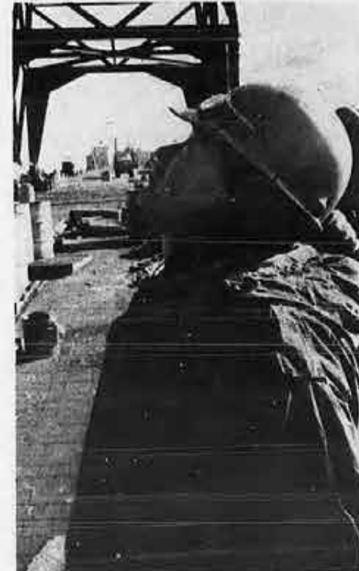
SIU-affiliated UIW member Max Reiter on the job at the former Brooklyn Navy Yard.
