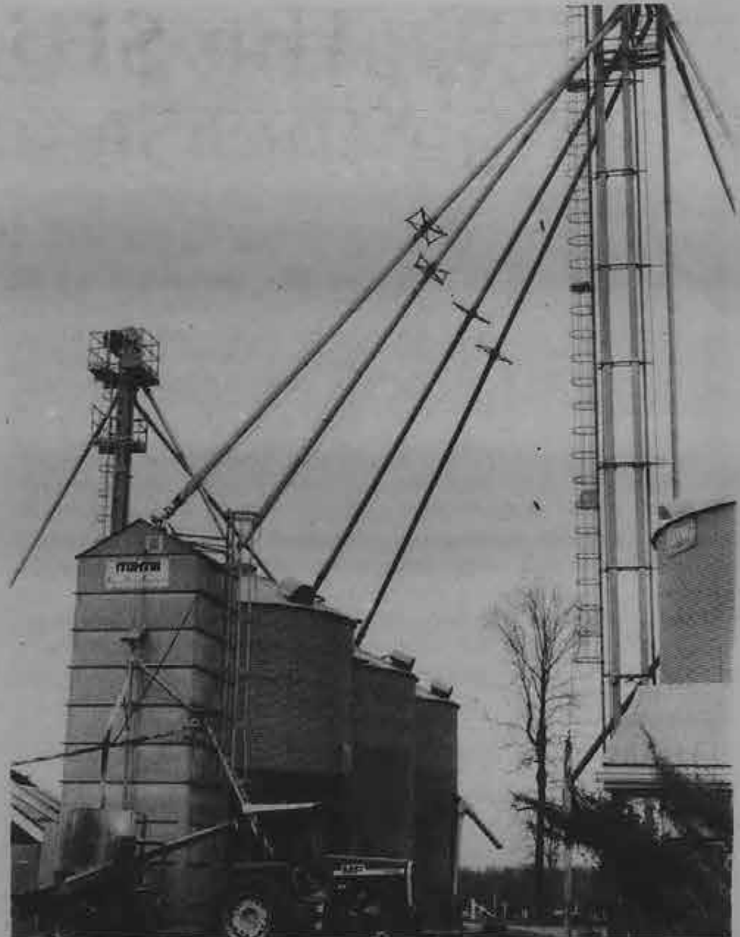
The five grain tanks are interconnected to the grain mill and each tank holds 80,000 bushels of corn.
