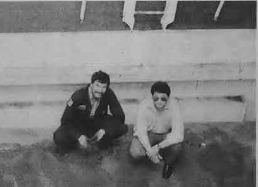
Inspecting the rusted container before it is removed are Bosun Charles Bowen (left) and Patrolman Rob Scrivens.
