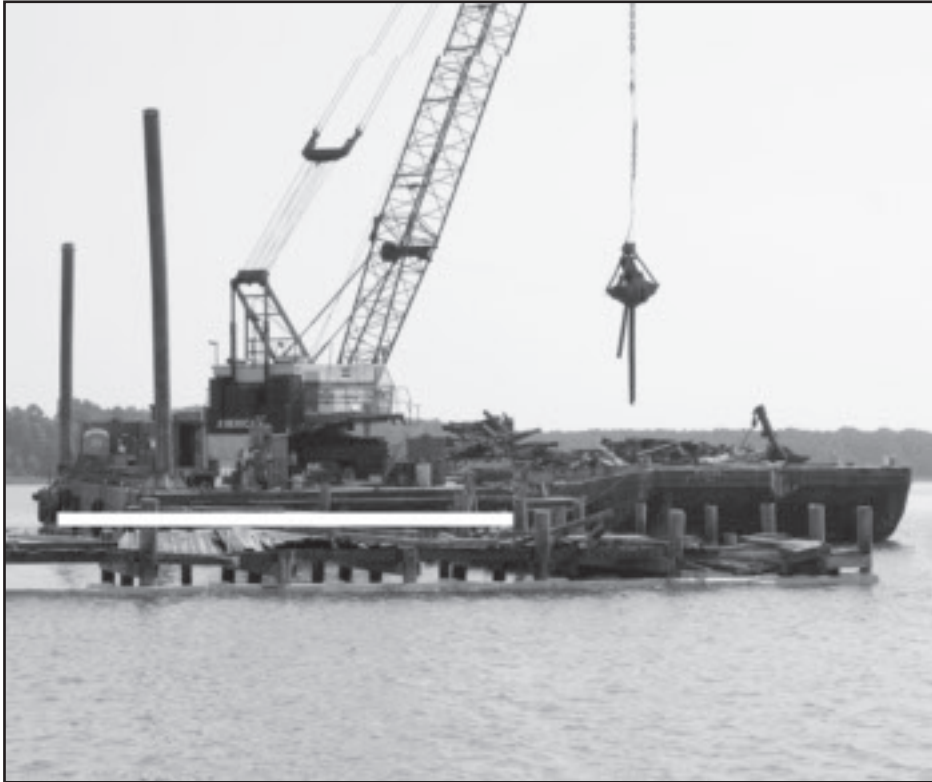
Early stages of the project include removing old piers and bulkheads, as shown in these two photos.
