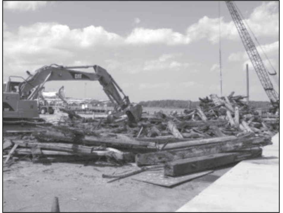
Early stages of the project include removing old piers and bulkheads, as shown in these two photos.
