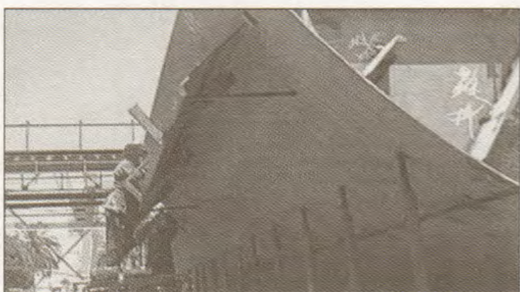
The first of two roll-on/roll-off ships for SIU-contracted Totem Ocean Trailer Express, Inc. is under construction in San Diego. It is scheduled for delivery in October 2002. For more photos of the early stages of the construction, see page 3.
