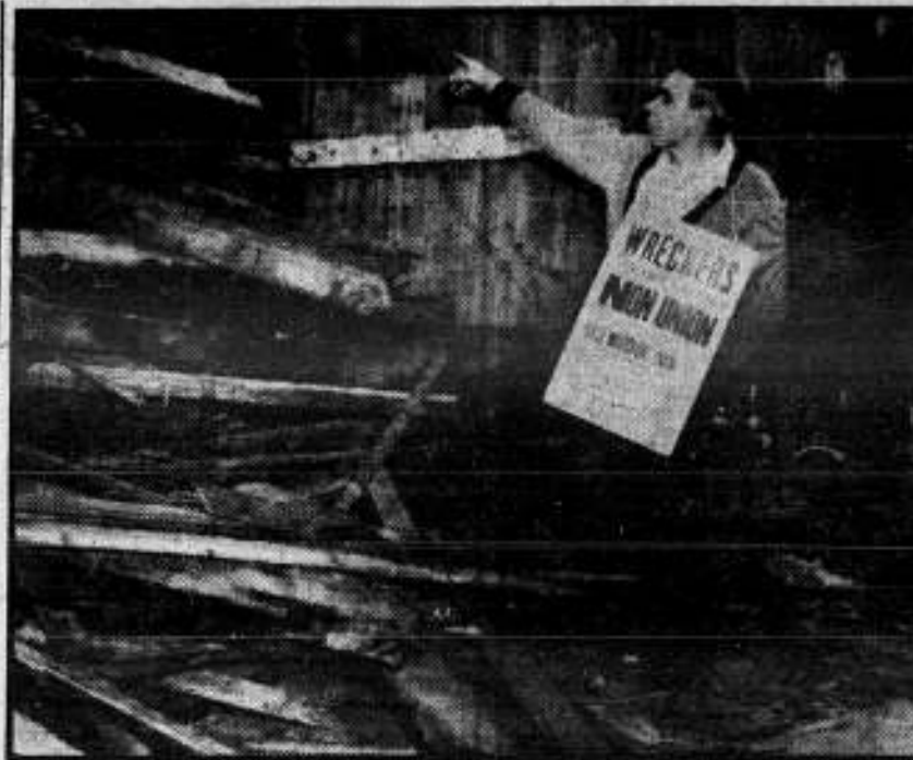
Ex-Seafarer William Frank points out collapsed house from which he pulled three non-union housewreckers while he was on picketline duty. Frank resumed picketing after the rescue.
