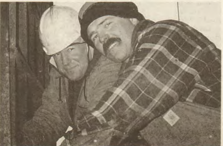
Dredgeman Randy Johnson (left) and Captain/Dredgeman Kevin Hollenbeck put bolts in place on the new bridge joint.
