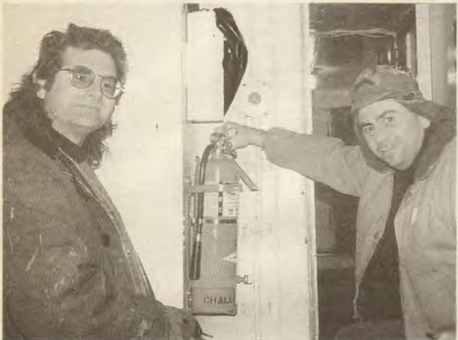
Mounting a new fire extinguisher in a passageway aboard the Medusa Challenger are Deckhand Michael Cushman (left) and Watchman Paul Bird.
