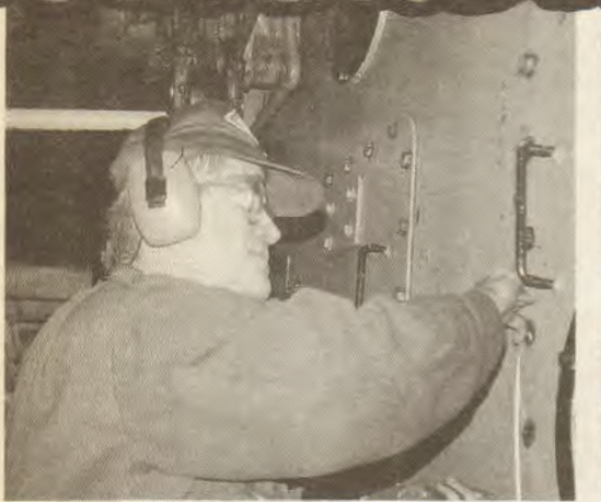
Installing gasket material for the Medusa Challenger is Oiler Dick Slade.
