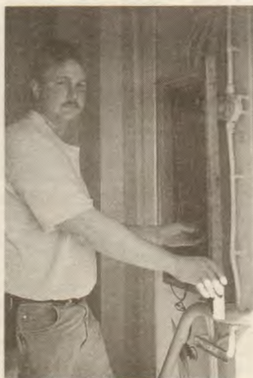
Checking a fuse box is QMED/Electrician John Miller.
