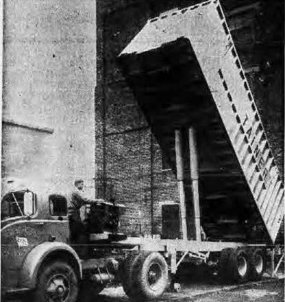
One man goes into action to show the ease with which the SIU-contracted Seatrain's new Tilt-Tainer can be off-loaded from a truck and set into its upright sile position. Platform on which the silo rests is in lower right corner of photo.
