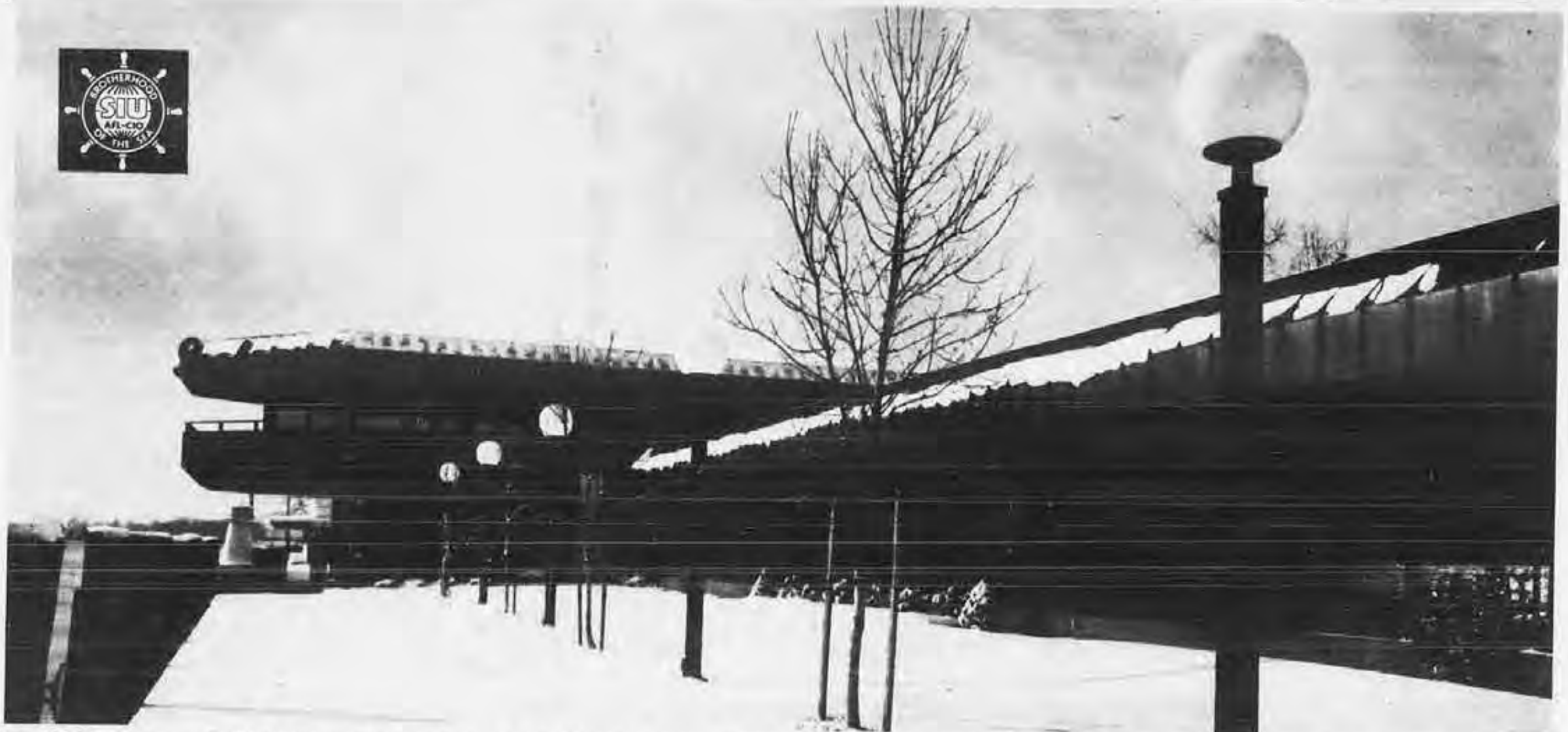
The Conference was held at the new Lakes Union Hall in Algonac, Mich. It took place in the second floor meeting room, which projects over the St. Clair River.
