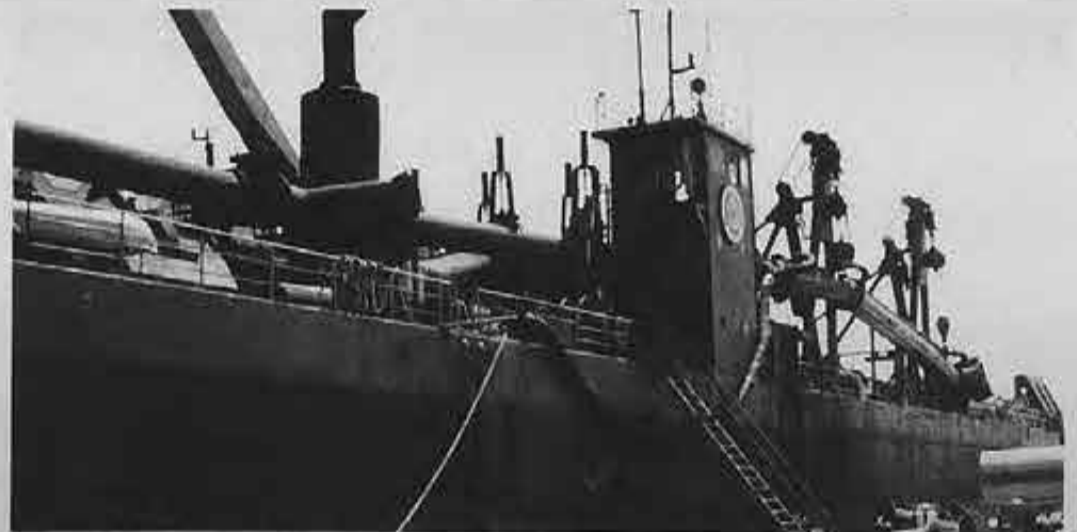
Pumping 15,000 cubic yards of sand on a daily basis, it took the dredge Long Island crew two-and-a-half months to restore sand to Maryland beaches.
