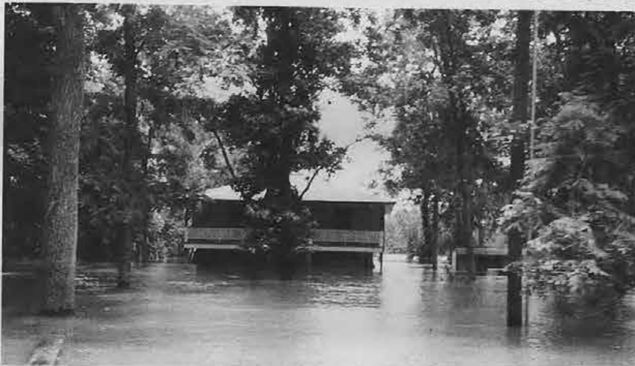
Electrician Jimmy Rogers has experienced four floods in five years, but this one was the worst, he said. The photo above shows the water level almost reaching the apartment he set up above his garage (foreground) and the top of the main house off to the right.
