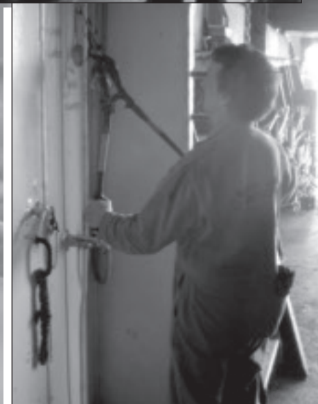
AB Dave Steele cuts old handles from a damper wire.
