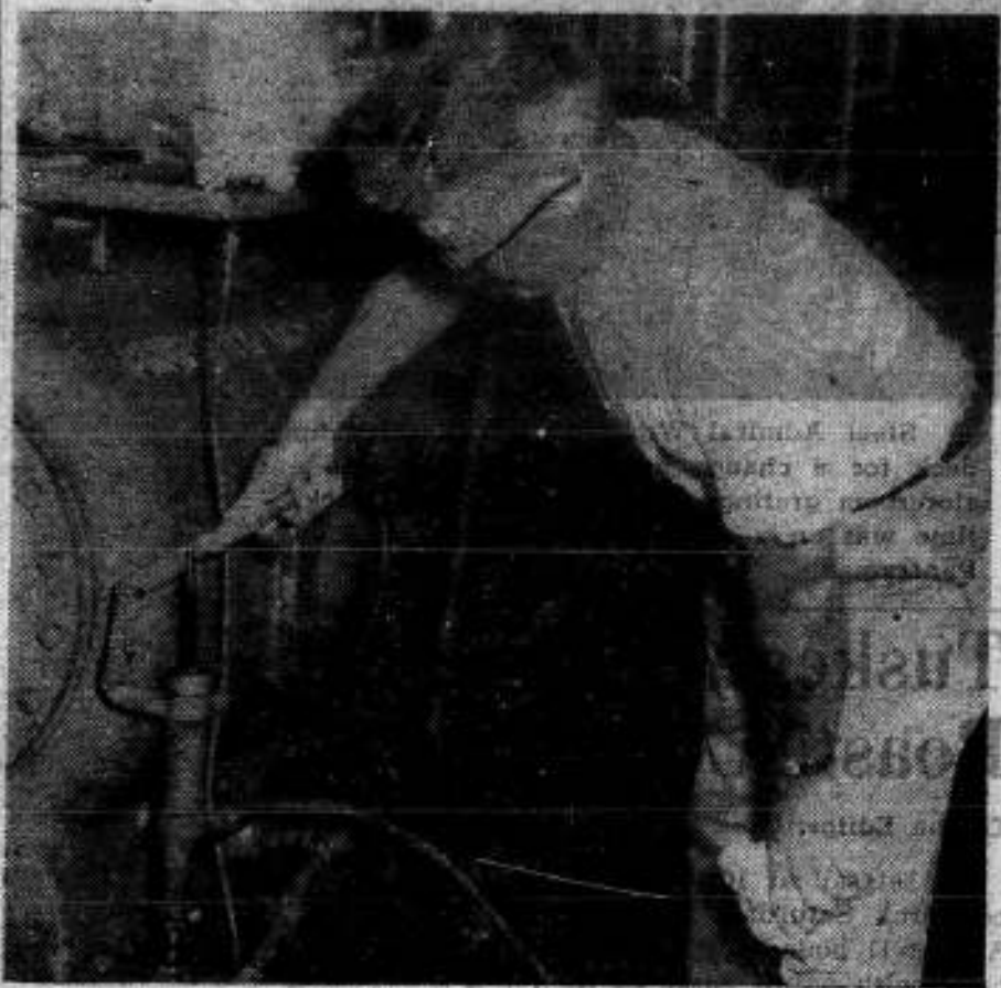
Reefer Engineer Jim Murphy takes a bit of oil from one of the compressors in the SS Puerto Rico's reefer room, wherein is located the ship's air-conditioning equipment. Jim is the ship's Delegate.
