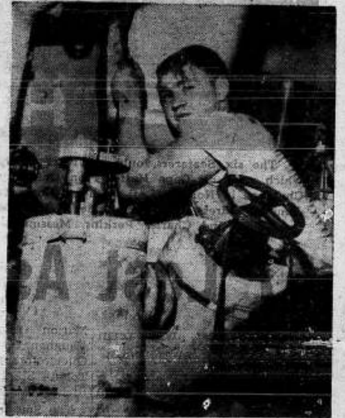
Jimmy Logan, Wiper, works up a sweat in a tight spot. He's busy replacing plates in a boiler casing, though he pauses a moment for Brother Beck's camera.
