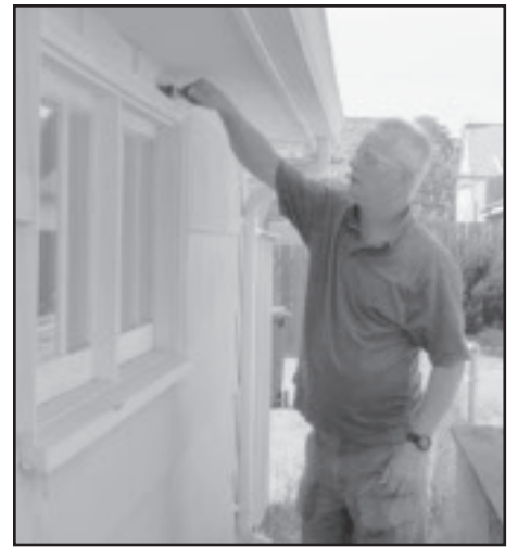
Electrician David Goodpastor removes old caulk
