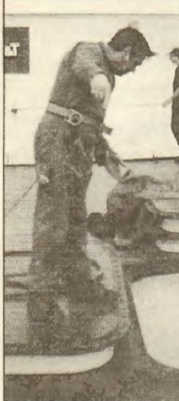
Directing crane operations on the deck of the cable ship is Bosun Jose Gomez .
