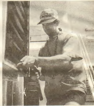
AB Walter Oswald takes careful aim to knock out a bolt in a vent.
