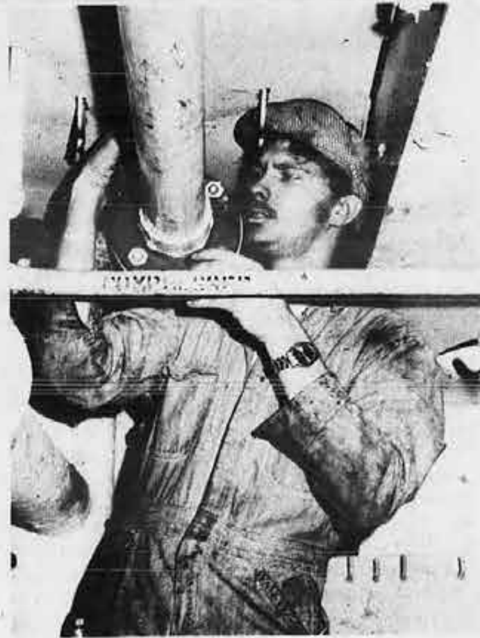
Third Engineer Carroll Knot repairs a pipe collar by sealing it.
